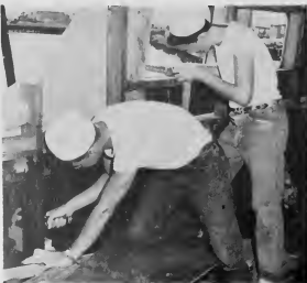
THE CABIN and other fittings are made of Surinam plywood, which is strong enough to match the teakwood hull. Tim Hagerty, right, and Artie Spitzer are working on window frames.
